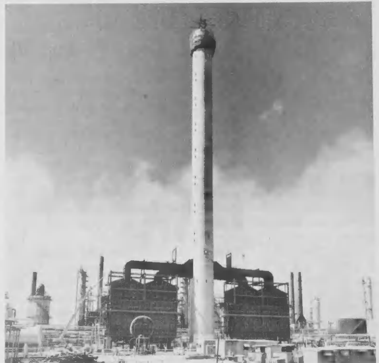
New furnace stack of Pipestills 5 and 6 nearing completion. Schoorsteen nobo pa fornu di Pipestills 5 y 6 biniendo cla.
